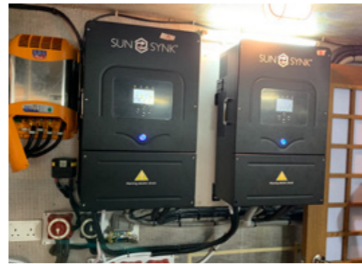
Two inverters wired together
