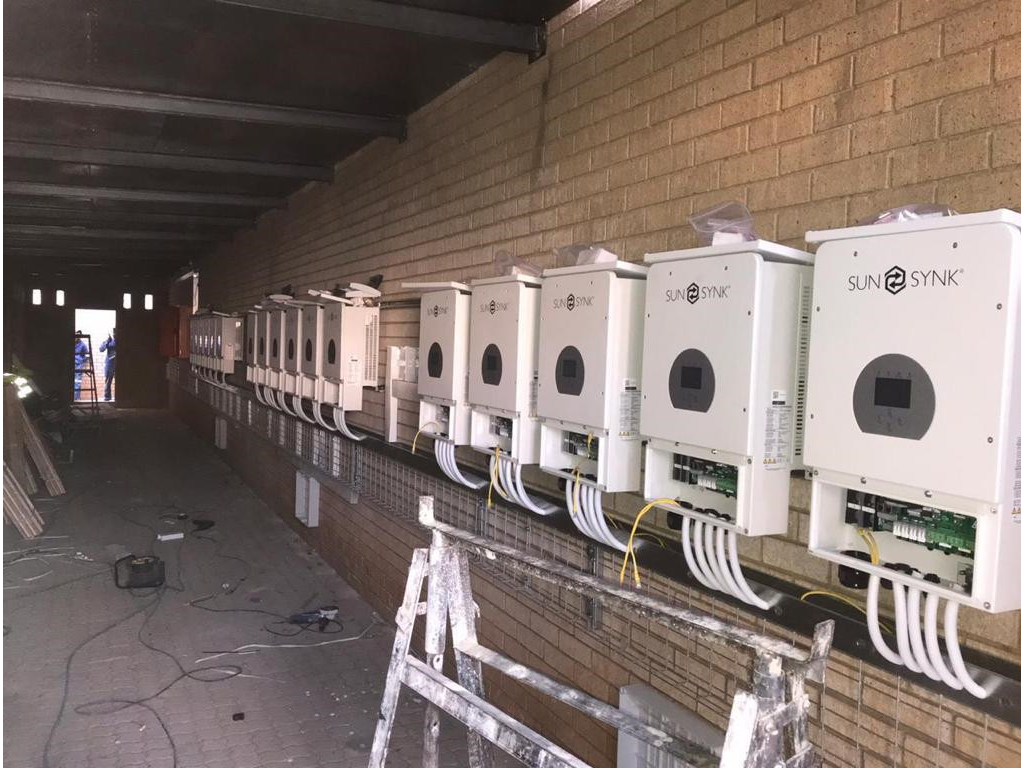
Figure 51 - Installation with many inverters.
