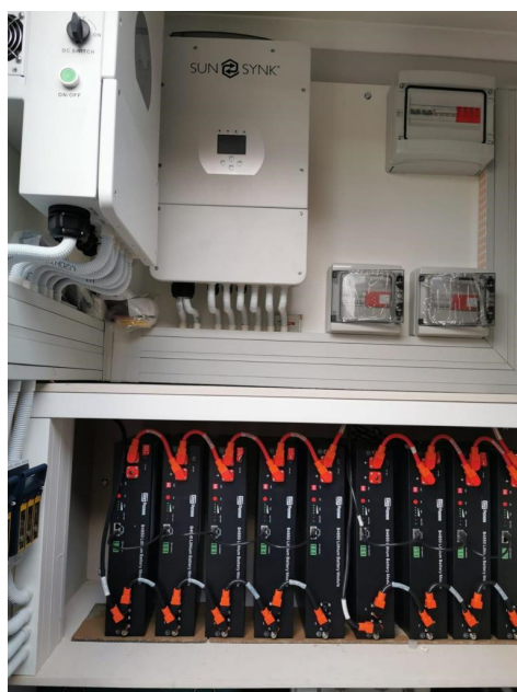
Figure 16 - Inverters with appropriate battery connections.
