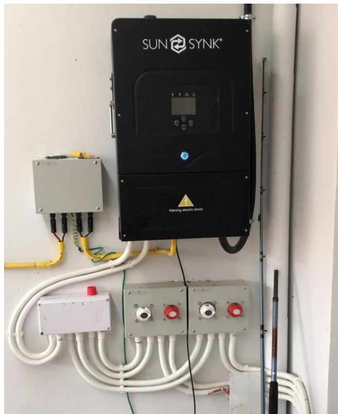
Figure 14 - Sunsynk inverter installation - black version.
