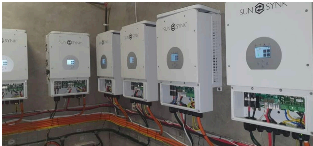
Figure 55 - Sunsynk inverters paralleled.
