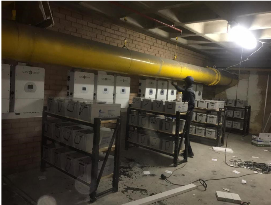
Figure 59 - Inverter installed in a dusty environment.
